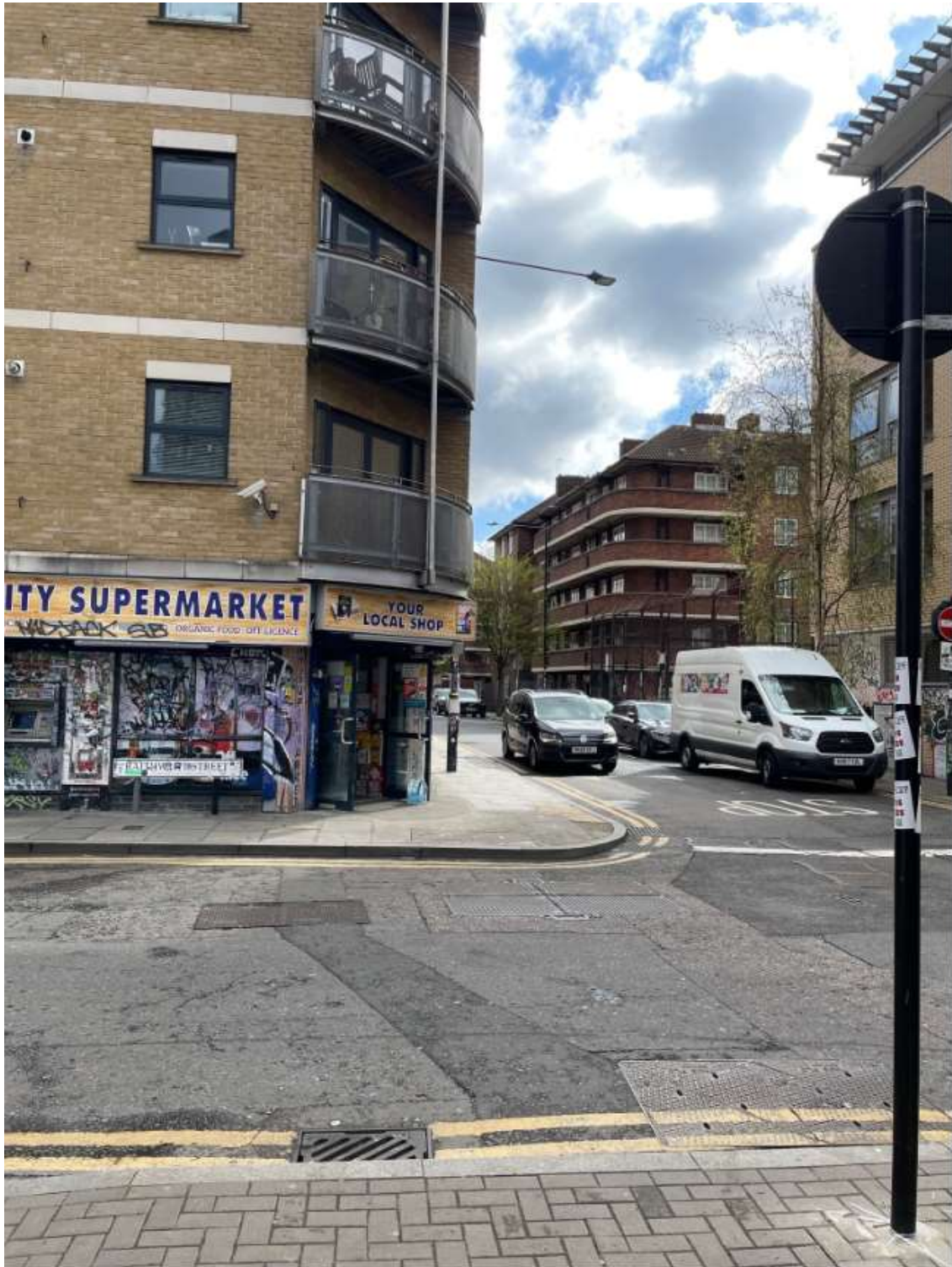
Premises photos: (Carwash), 1 Quaker Street, London E1 6SZ
